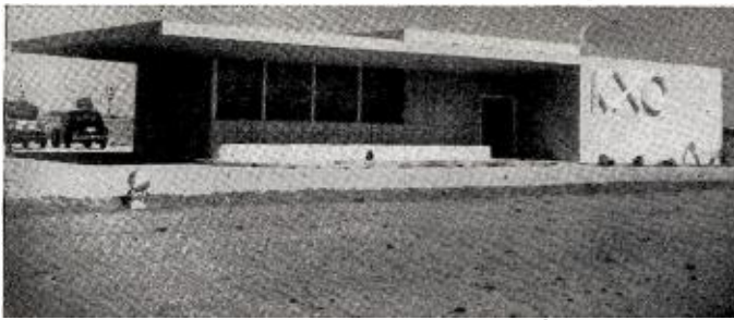
RANCH STYLE is design of new modernistic studio and office building for KXO El Centro, Calif., which celebrates its 20th birthday this year. Modern in design, building contains no windows with all ventilation controlled through concealed ducts and vents. Doyle Osman is the station's general manager
